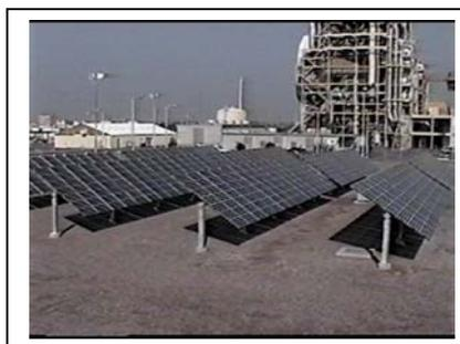
The SolarTrak® Controller uses mathematical computation for the Sun's position in the sky and counts electronic pulses (feedback) to determine the actual array (moving part of the solar tracker) position. By making these two positions coincide on a continuous basis throughout the day it will cause the array to follow the Sun.
