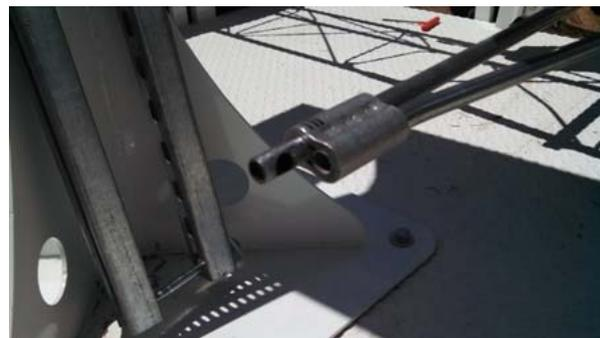
The wind direction vane goes on the same side as the storage box. Slide the connector on to the strut and tighten the set screw while lightly wiggling the instrument bracket to fully seat the screw in the hole provided. The anemometer cups go on the other side. Wrap each instrument wire loosely with the same 4" droop loop around each strut and direct the wires down the same path inside the tower as the other wind instruments.
