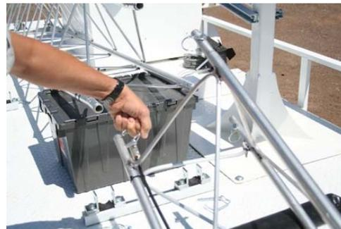
Systematically, in a circular pattern, push in one upright at a time while maintaining pressure on the other two uprights to prevent them from backing out... rotate around, a little at a time until you can get a screwdriver in one hole... then it gets easier...
