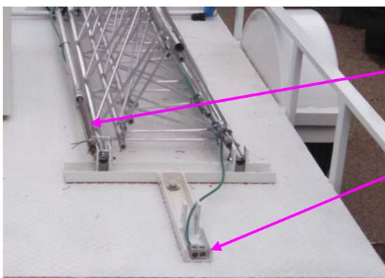
Sink the included eight-foot grounding rod within two feet of the rear of the trailer then connect it to the connector at the back of the hinge plate.
